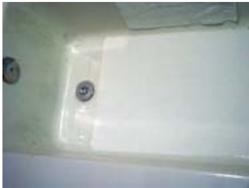
Rebuilt and Slip-Grip coated
